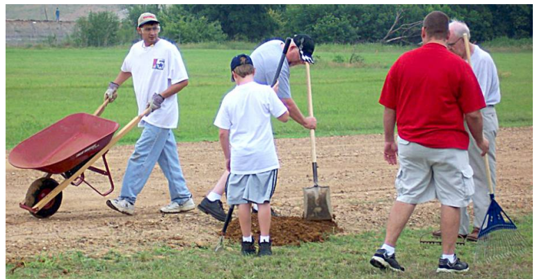
Workers prepare the runway for laying of the petra-mat.
